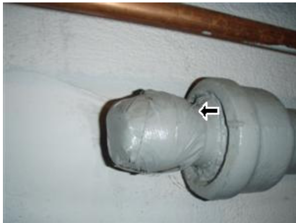
4.0 Picture 1 properly seal
