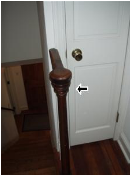
8.3 Picture 1 tighten rail
