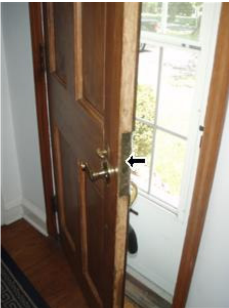
2.1 Picture 1 repair lock
