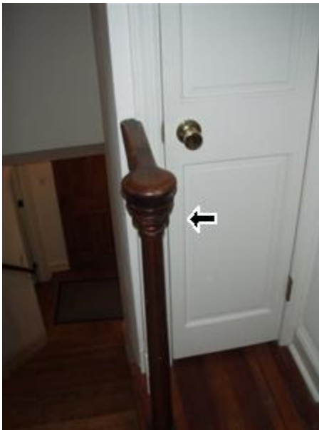
8.3 Picture 1 tighten rail
