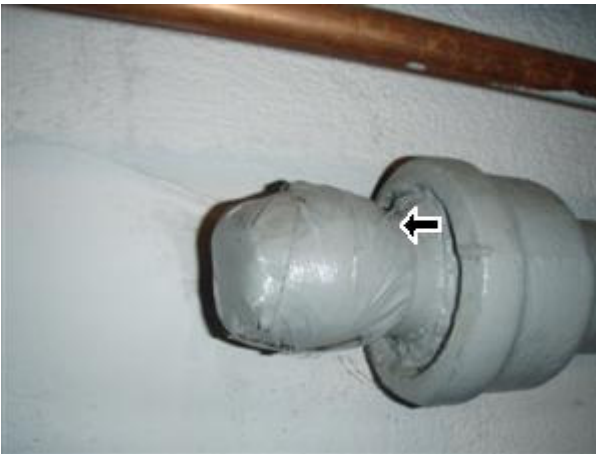
4.0 Picture 1 properly seal
